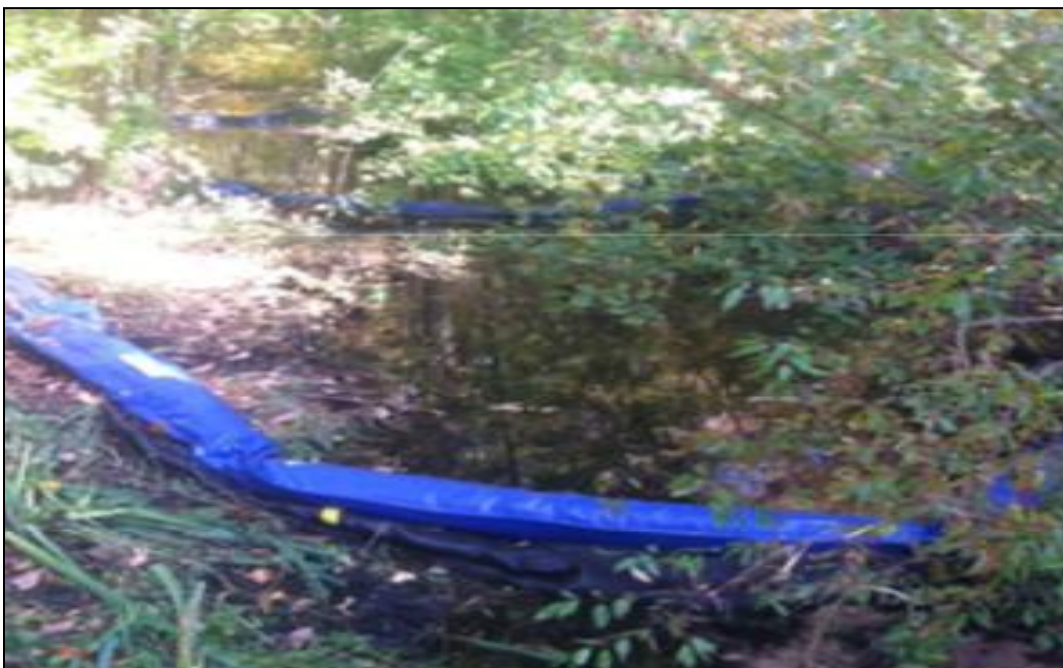
Figure 68. A tributary filter strip (photo courtesy of Lake Savers, LLC).
