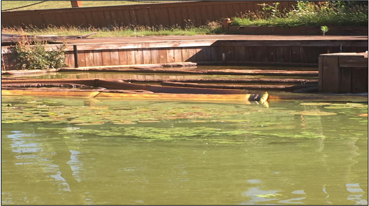
Figure 8. An oil boom in place to reduce oil seepage from a property in Fenner's Ditch (RLS, 2017).
